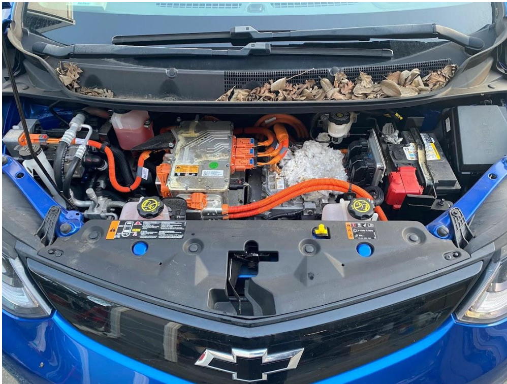
Not a District vehicle, but a reminder that electric vehicles can provide warm nesting locations for rodents.
