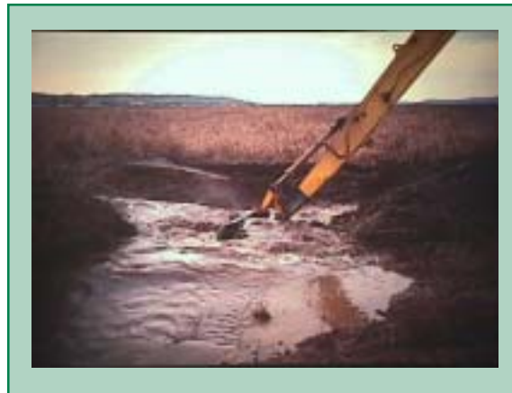
An excavator hard at work clearing an overgrown marsh channel
