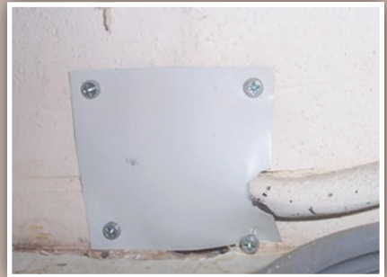
Power supply hole sealed with metal flashing.*
