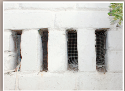
Check for loose mesh in foundation vents.
