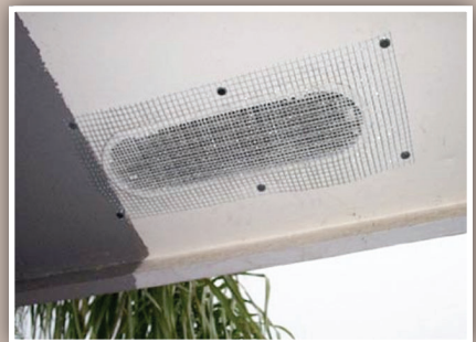
Soffit vent hole sealed with screen.*
