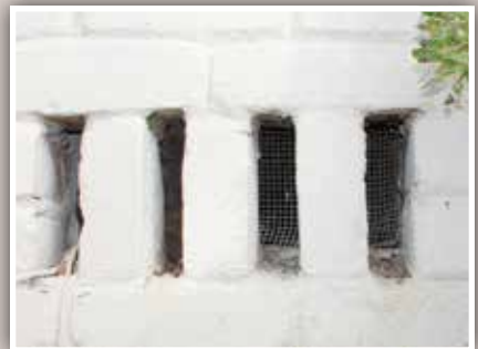
Check for loose mesh in foundation vents.
