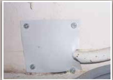
Power supply hole sealed with metal flashing.*
