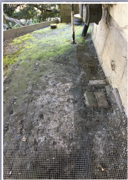
Above ground screening using concrete screw anchors and galvanized garden stakes
