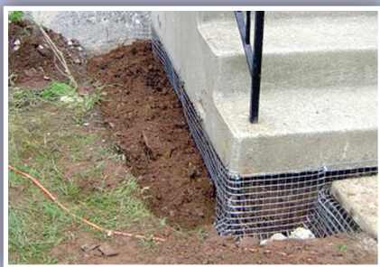
L-Shaped screen application around foundation**
