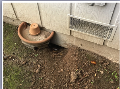
A hole beneath foundation is evidence of a skunk burrow
